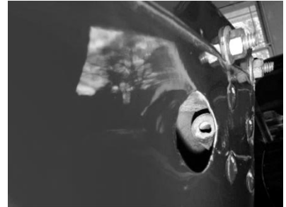
Lanyard passes through tube inside door; plunger and coil spring retract into tube from jamb side to allow door to open
